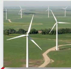
Langdon Wind Energy Center Langdon, N.D.
