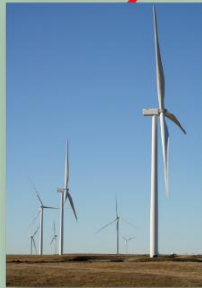
Oliver III Wind Farm Center, N.D.
